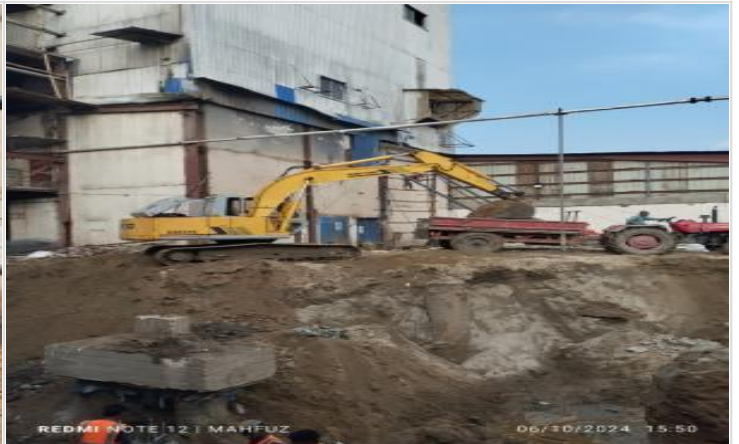
Earth Excavation on 06-10-24
