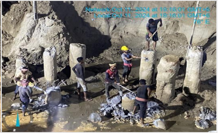
Pile head breaking on 11-10-24
