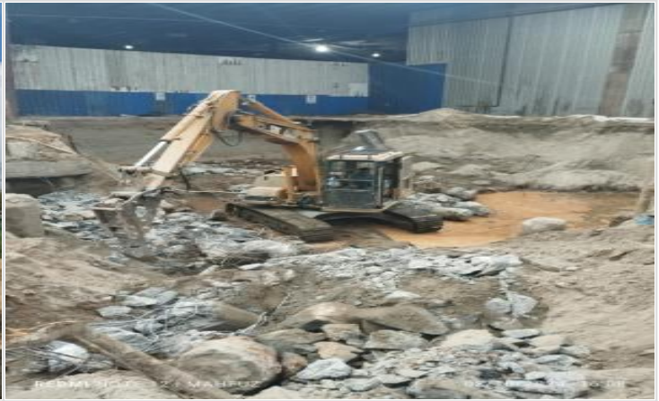
Dismantling by hydraulic breaker on 08-10-24
