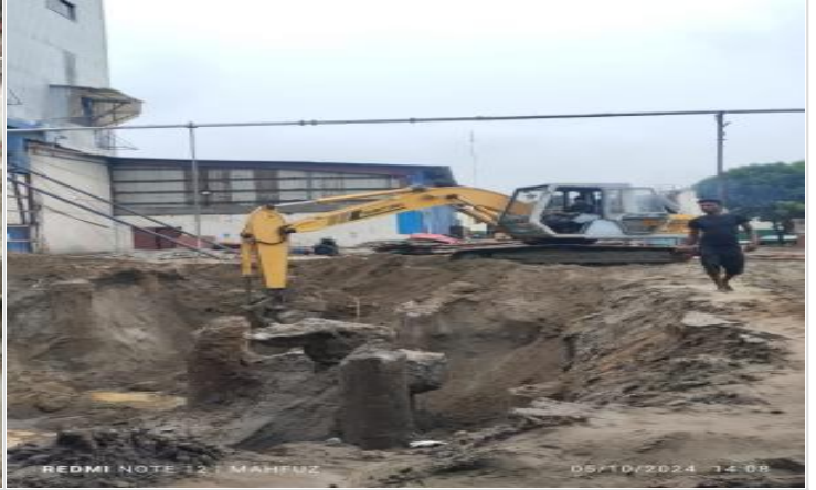
Earth excavation on 05-10-24
