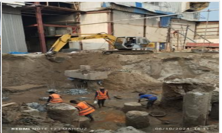
Pile head breaking on 07-10-24
