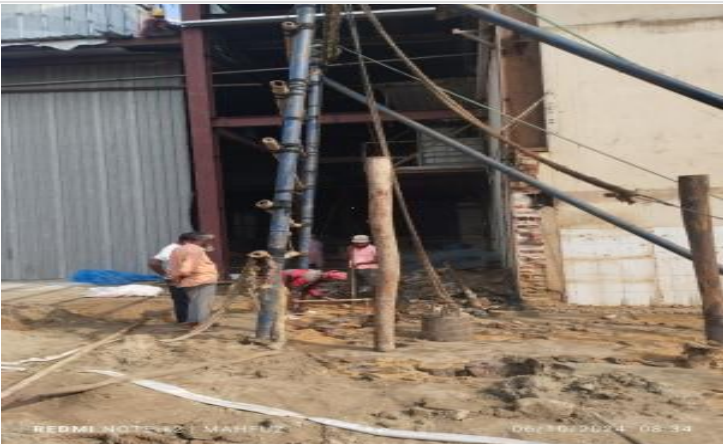
Wooden shore pile driving on 06-10-24
