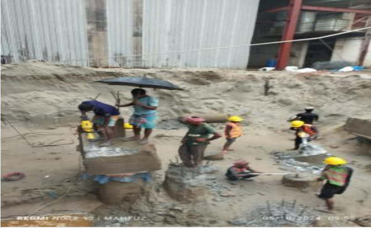
Old base breaking on 05-10-24
