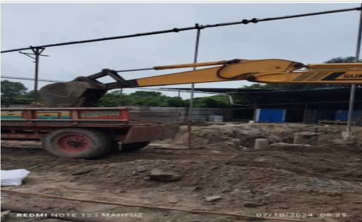
Earth excavation on 07-10-24
