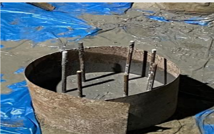
Pile Load Test-PDA-Pile Development on 10-10-24
